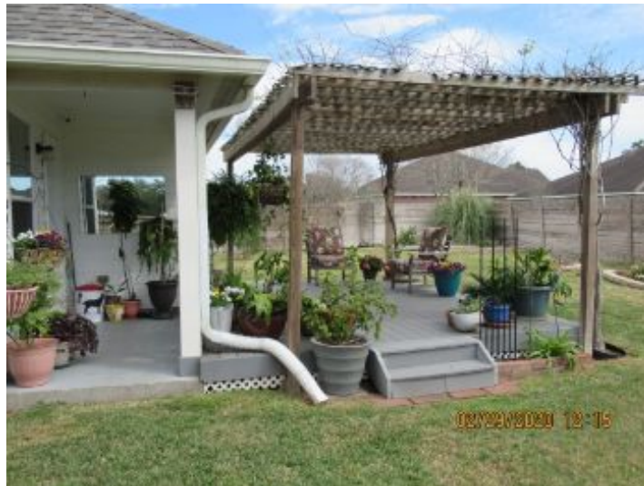
This is a good picture showing the patio cover is not attached to the home nor is the deck. Both appear to function as intended at the time of the inspection.
