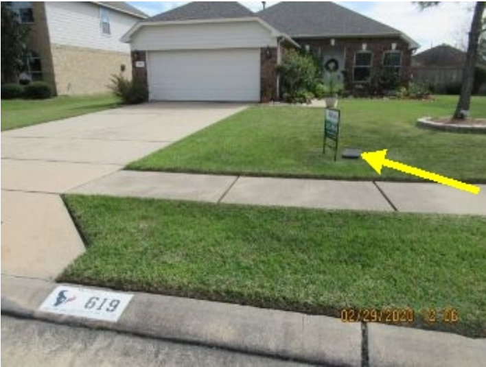
Water meter location.
